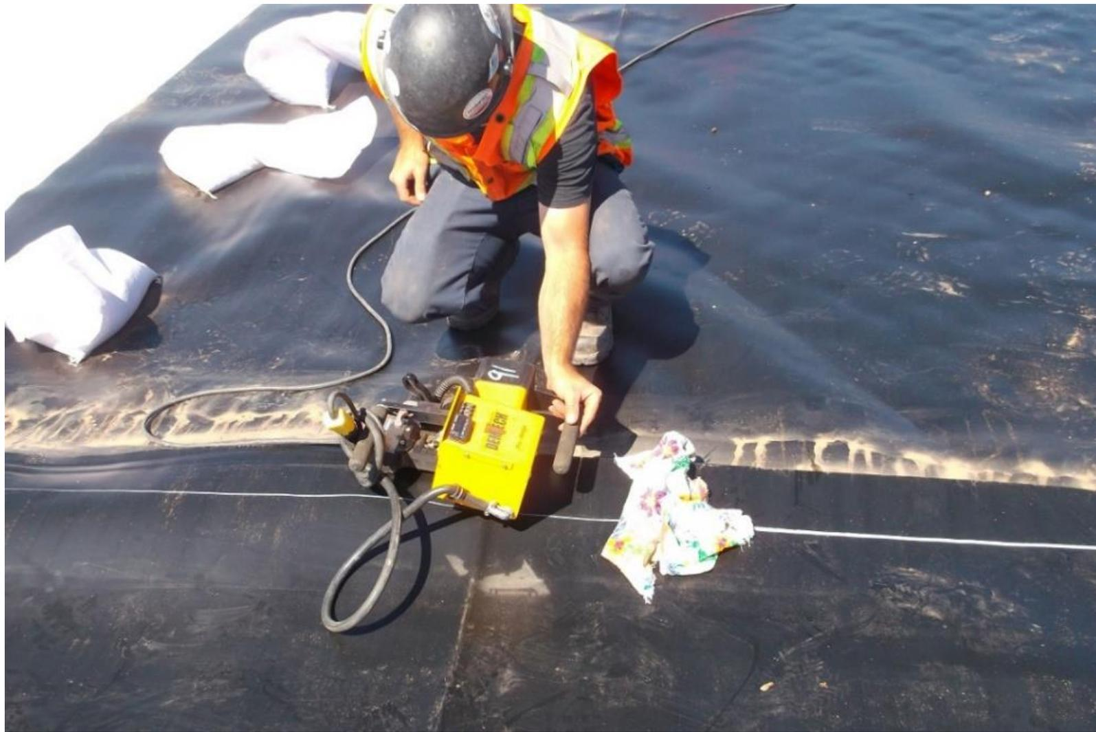
Representative Landfill Construction – Place geomembrane liner over recompacted low hydraulic conductivity soil base liner. Geomembrane is typically 80 mil HDPE. NOTE – wrinkles in liner; degree of wrinkles can vary widely but is important!!
