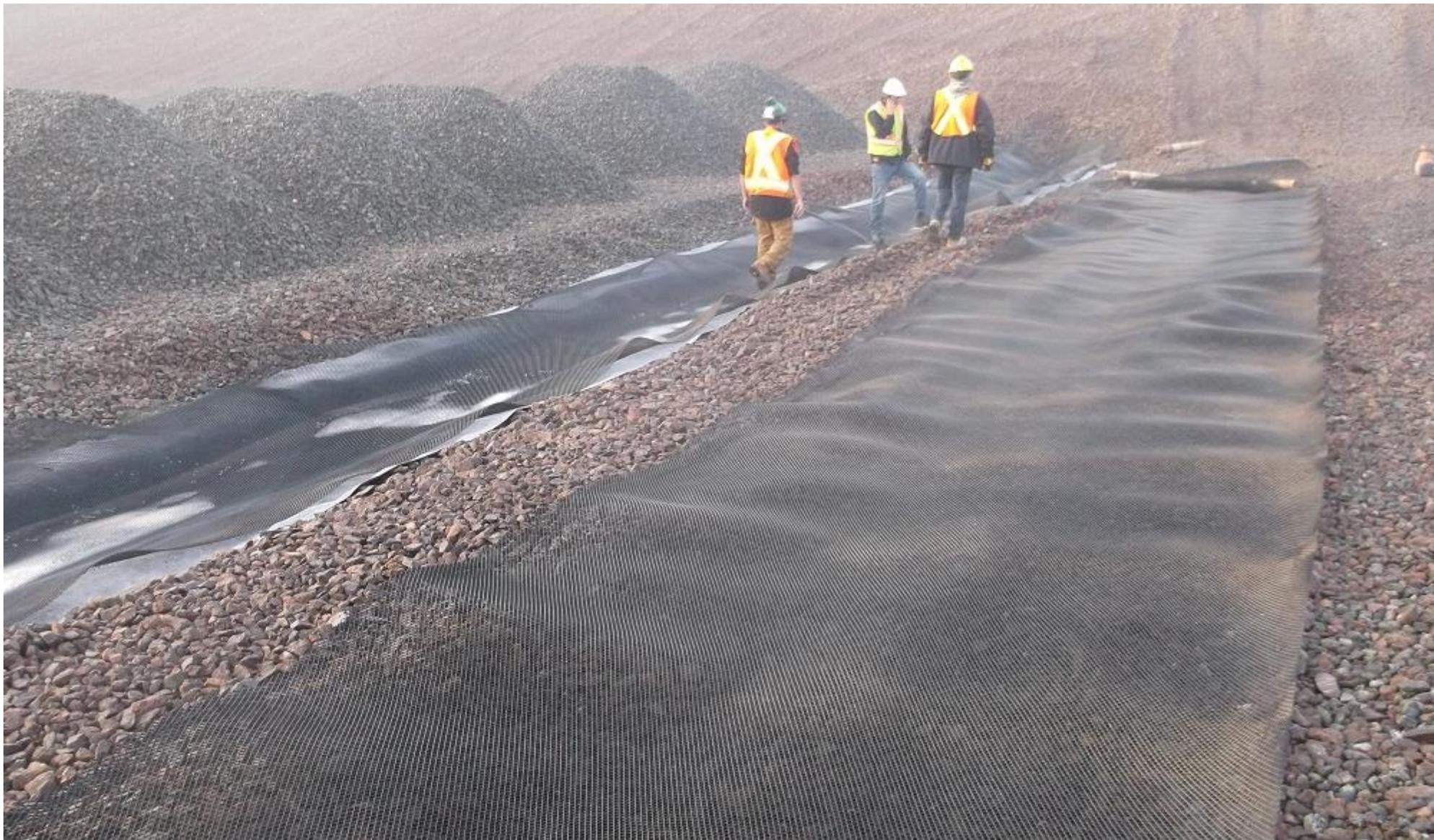
Representative Landfill Construction – Place drainage layer and piping (not shown) for leachate collection.
