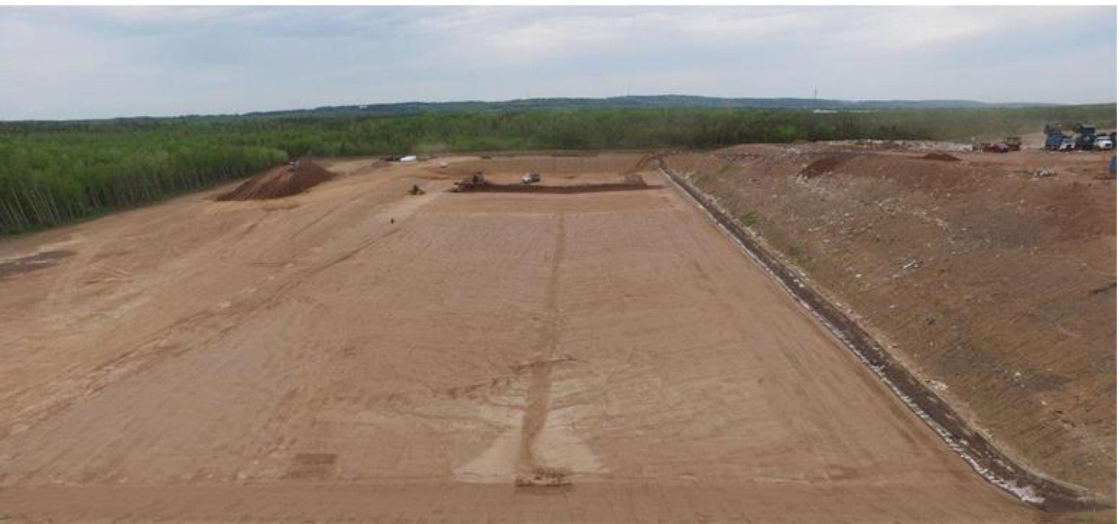
Representative Landfill Construction - Excavate and prepare subgrade (and place underdrain layer, if applicable), place and compact low hydraulic conductivity soil base liner prior to geomembrane liner construction.
